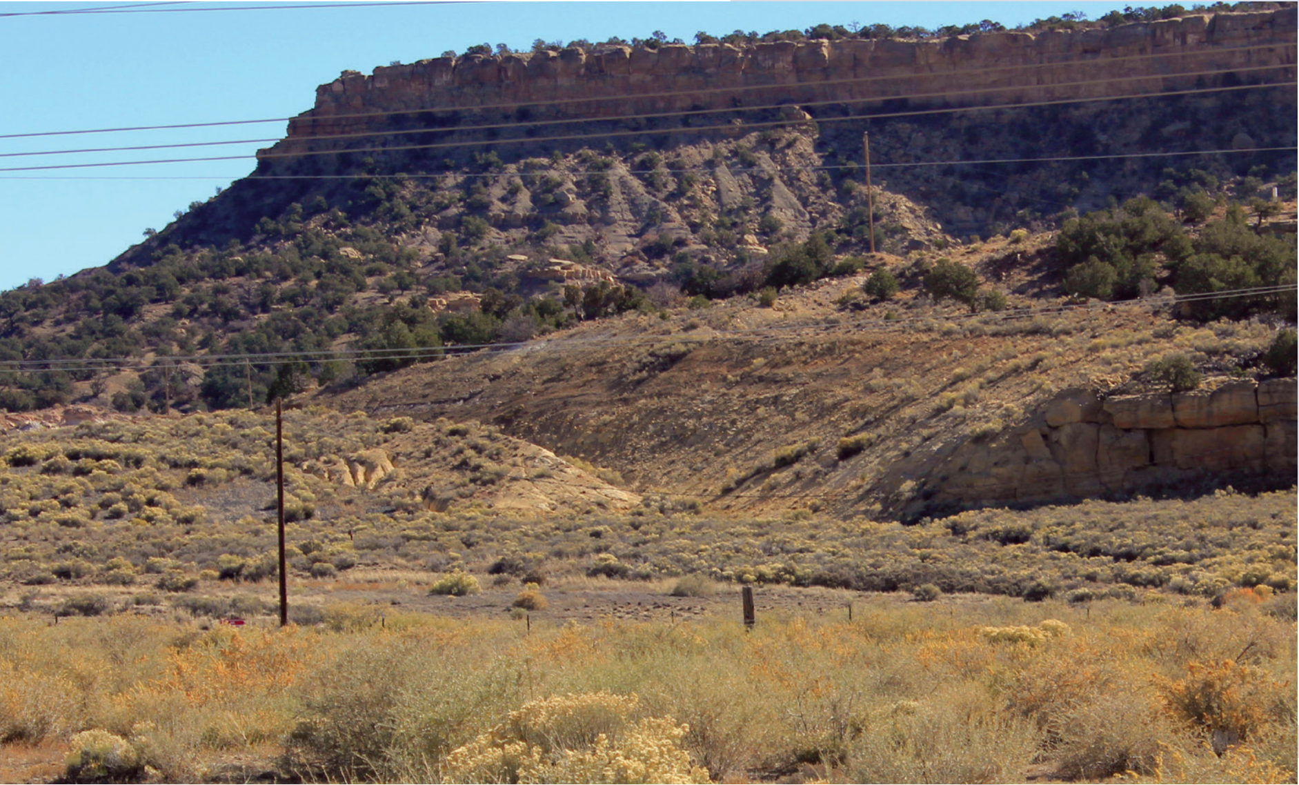
The tailings dam spill on July 16, 1979 was the largest release of radioactive contaminants in the history of the United States. More than 1,000 tons of radioactive waste and 360 million liters of contaminated effluent entered the Puerco River. Photo: © Rose Jenkins
