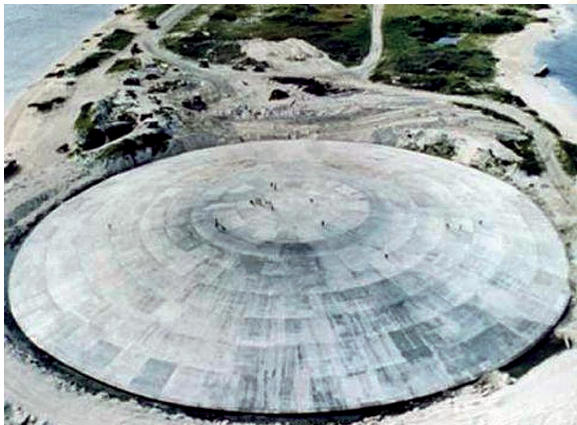
After nuclear testing had ended, part of the Runit Island (Enewetak) was so badly contaminated that an eight meter high concrete sarcophagus was erected to seal it off. Photo: © U.S. Defense Special Weapons Agency
