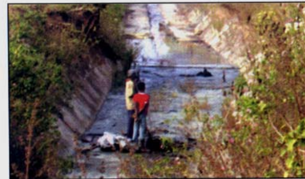
Leakage site tailing pond Jadugoda
